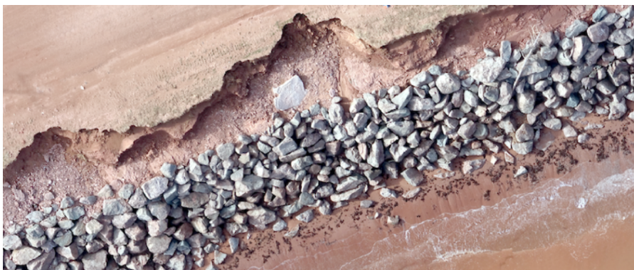
Figure 10- Example of overtopping erosion at armourstone revetment - Source: UPEI
